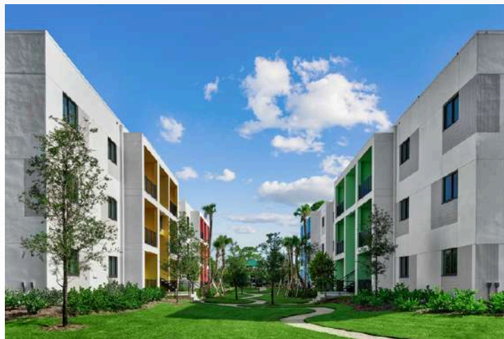
A small crew of unskilled workers built this four-building, 96-apartment complex in Palm Springs, Florida (All images courtesy of Renco USA)
