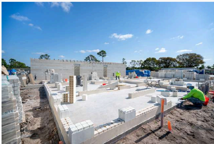
Each 3-storey block was built by 11 unskilled workers equipped only with a mallet and glue gun
