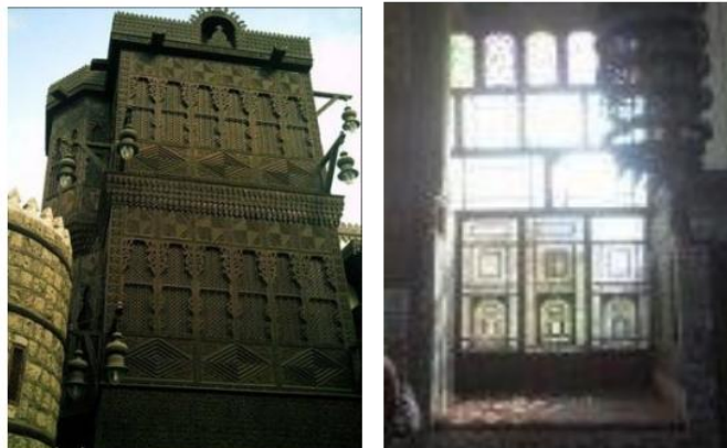
Figure (5), Illustrates How Al-Mashrabia controls air and natural light in addition to provide privacy.
