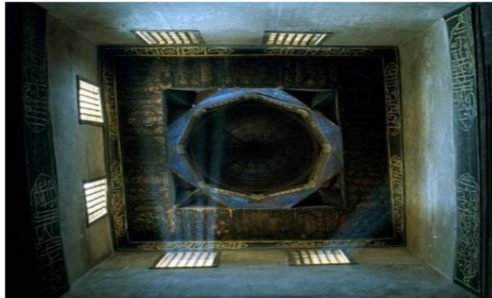
Figure (4), Illustrates how Al-Shokhshikha provides ventilation and indirect lighting
