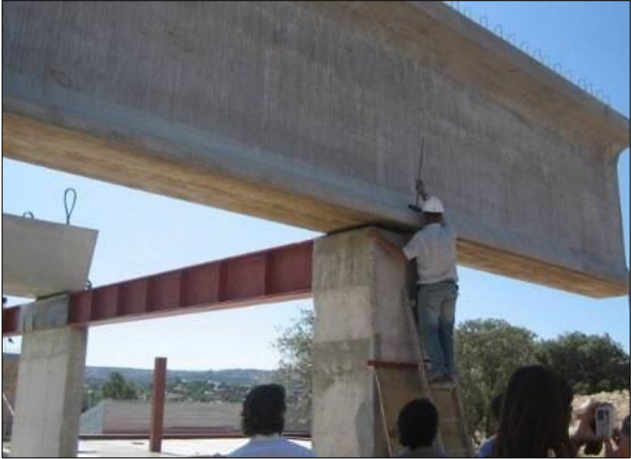
Simple Support in a Structure
