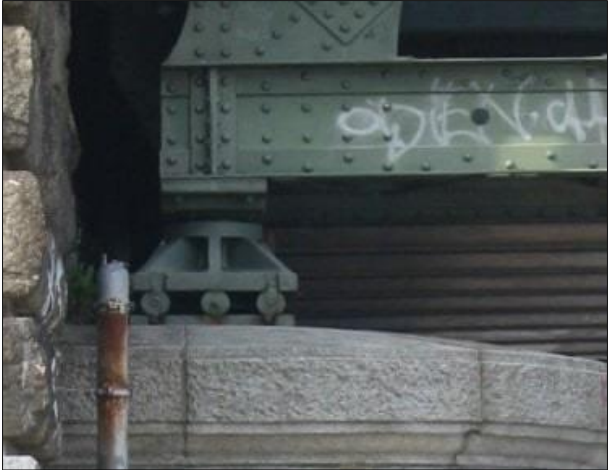
Hinged Support in a Structure
