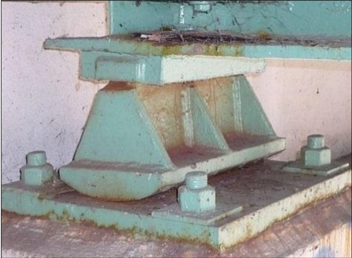
Rocker Support in a Structure
