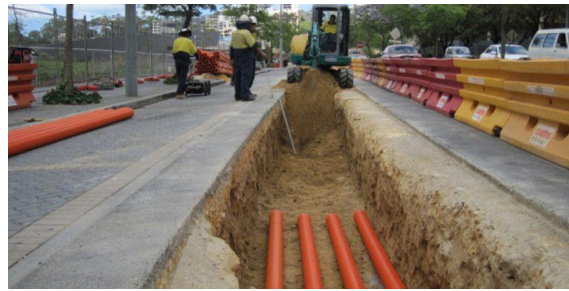
Figure 4: underground burial cables activities
